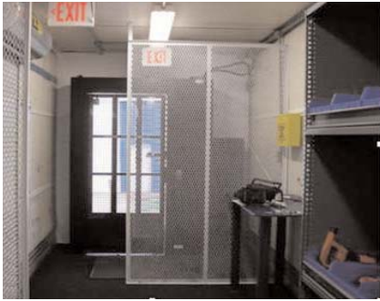
Inside the trailer looking towards the portal. Notice the RF Shielding fences on the right and left
