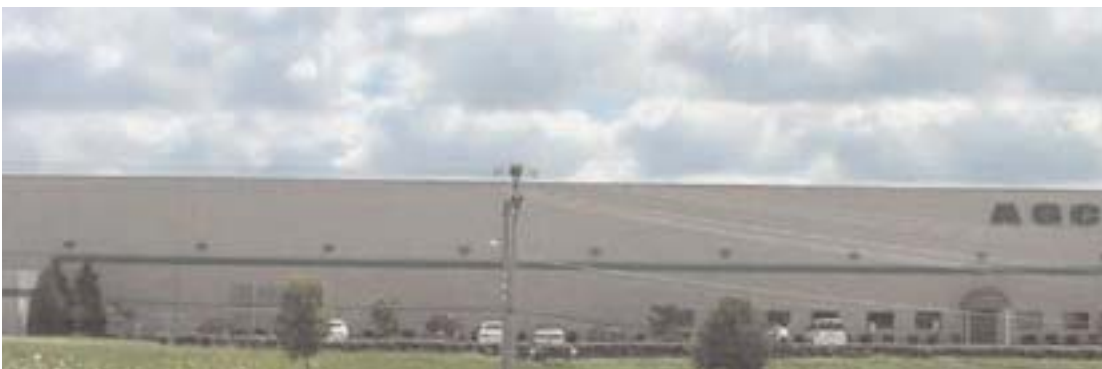
AGC's facility located in Winchester, KY
